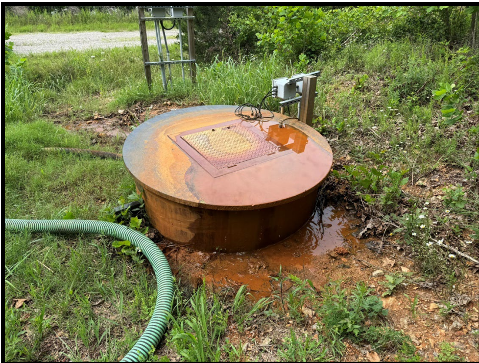
Photograph 2: View of VLCS-1 sump at capacity.
