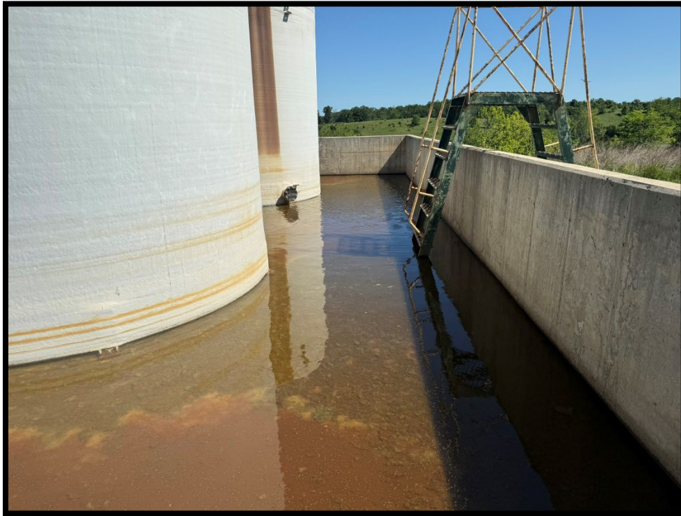
Photograph 3: View of leachate tank containment.
